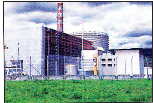
Fig. 3.16 : Nuclear power station, Kalpakkam
