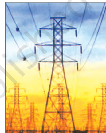
Fig. 3.7: National Power Grid to supply Electricity
